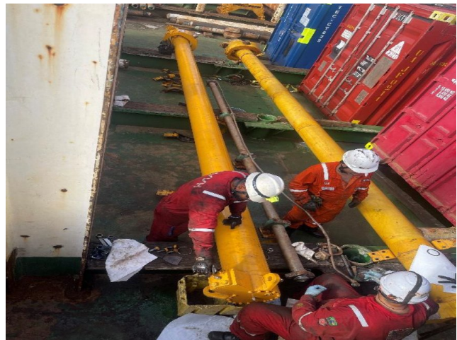
Figure 4 — LMI technicians handling and positioning catwalk hydraulic cylinders reassembly aboard the West Tellus
