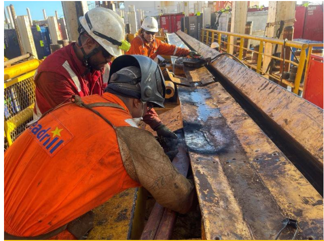
Figure 2 — LMI crew conducting close inspection and mechanical work on the Pipe Catwalk rail assembly
