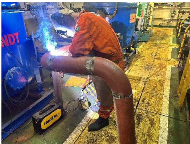
Figure 10 — LMI welder performing pipe modification and connection work on the degasser suction and discharge lines
