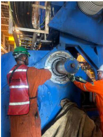
Figure 5 — LMI technicians performing disassembly and bearing removal on the mud pump crankshaft end during overhaul
